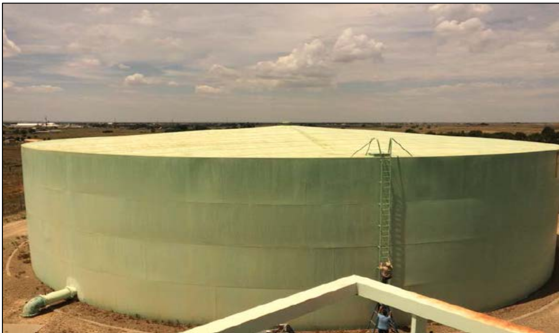
City of Portales Johnson Hill Tank Battery
